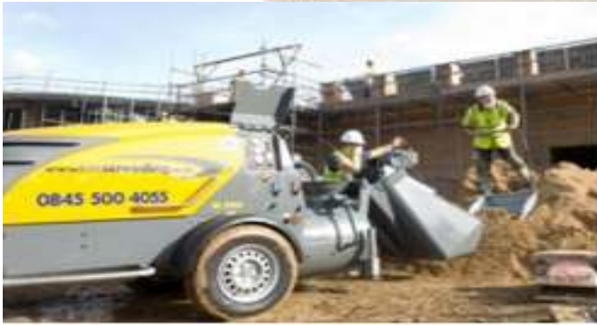
Fig 2 Cement screed Mechanical mixing
