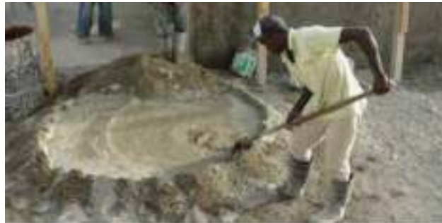
Fig 1. Cement screed hand mixing
