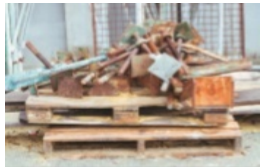
Figure 5.1 un clean work area
