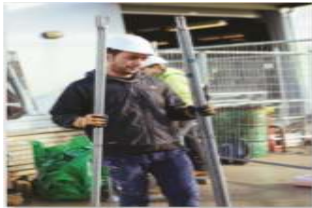
Figure 2.6.1 Erecting framed scaffold
