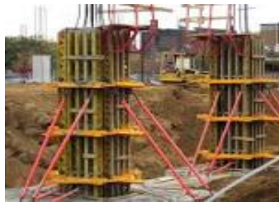
Fig 2.4.-:Bracing of column
