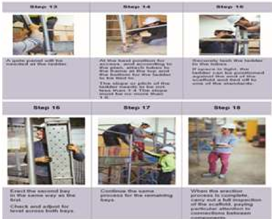
Fig 2.1 9:- Steps erecting framed scaffold
