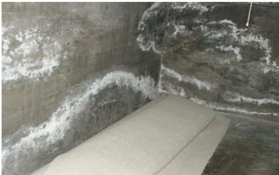
Fig3.7 Efflorescence
