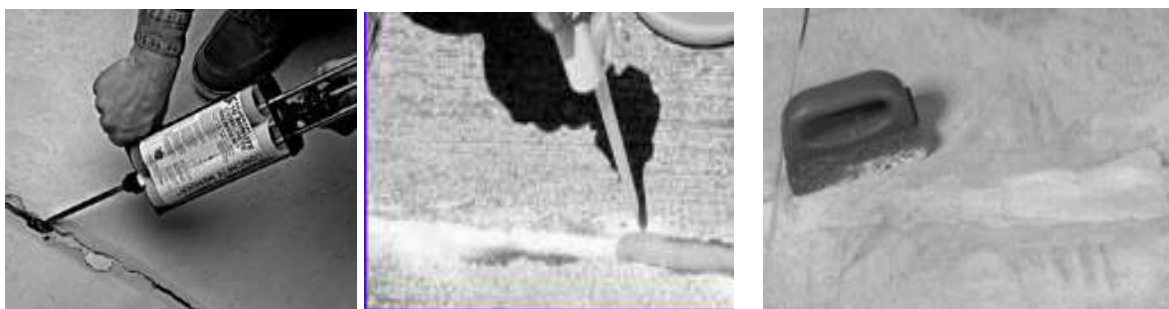
Fig.2.8. Epoxy concrete repair
