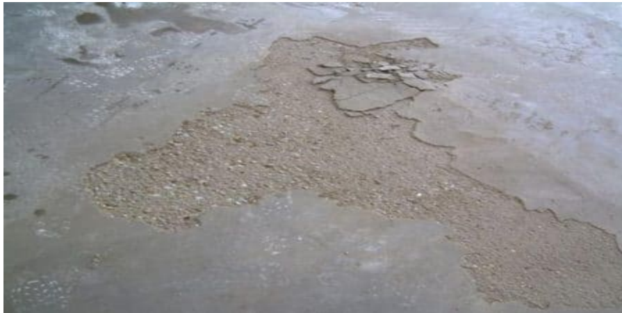
Fig3.4 Delamination
