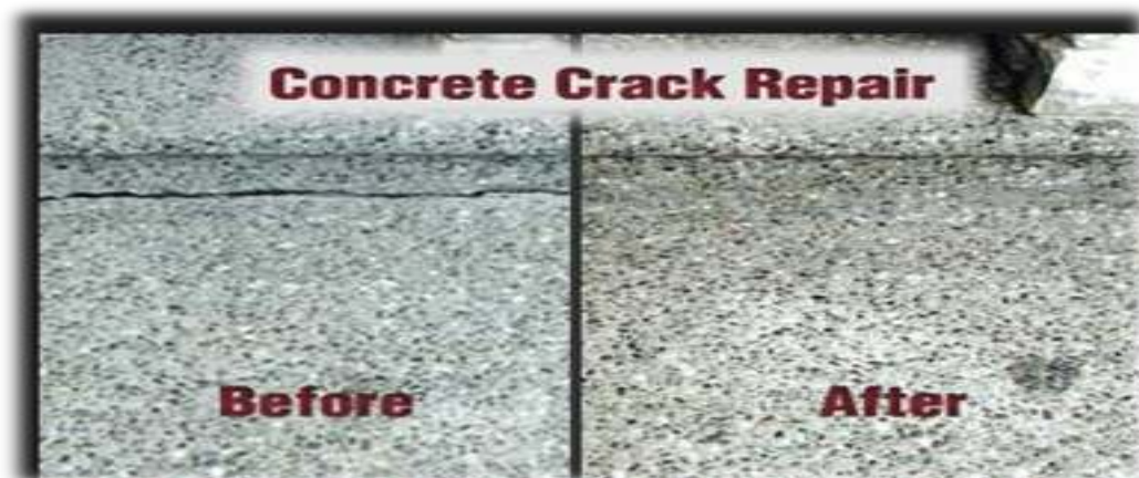
Fig.2.7. Concrete crack repair
