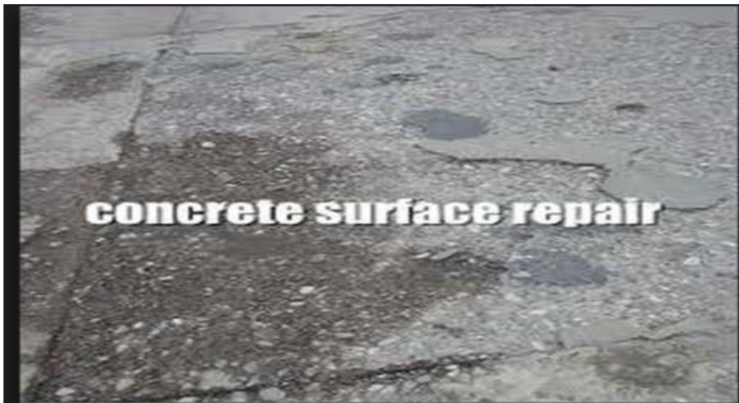
Fig2.2 concrete surface repair
