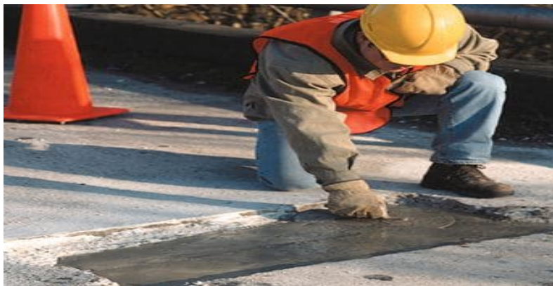
Fig3.11: Quick-set Non-shrinking Mortar
