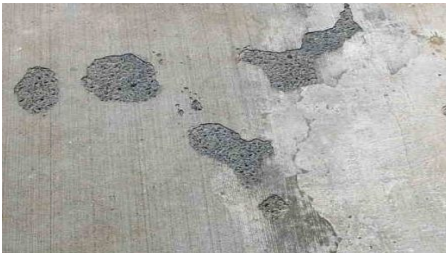
Fig3.3 concrete blistering
