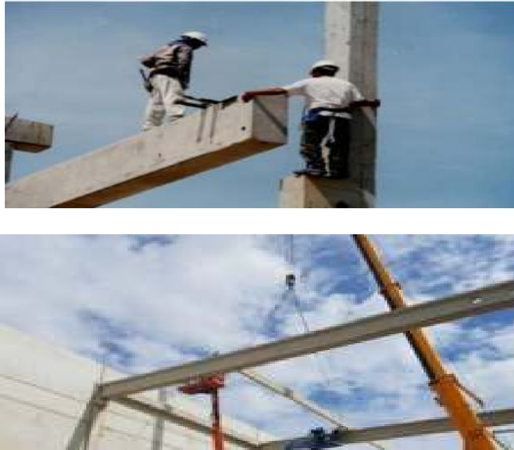
Fig.2.18.Precast Beam and Girders
