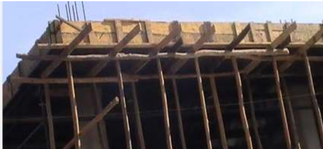
Fig.1.23. Beam and Slab Formwork
