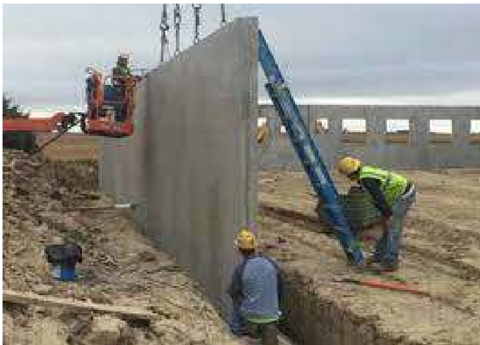
Fig. 3.3b: Fixing positioning for precast cladding
