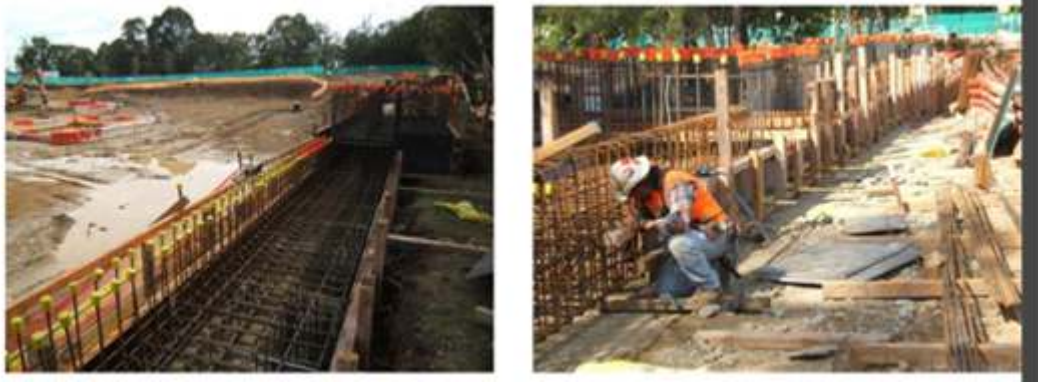
Fig1.20.Beam Formwork
