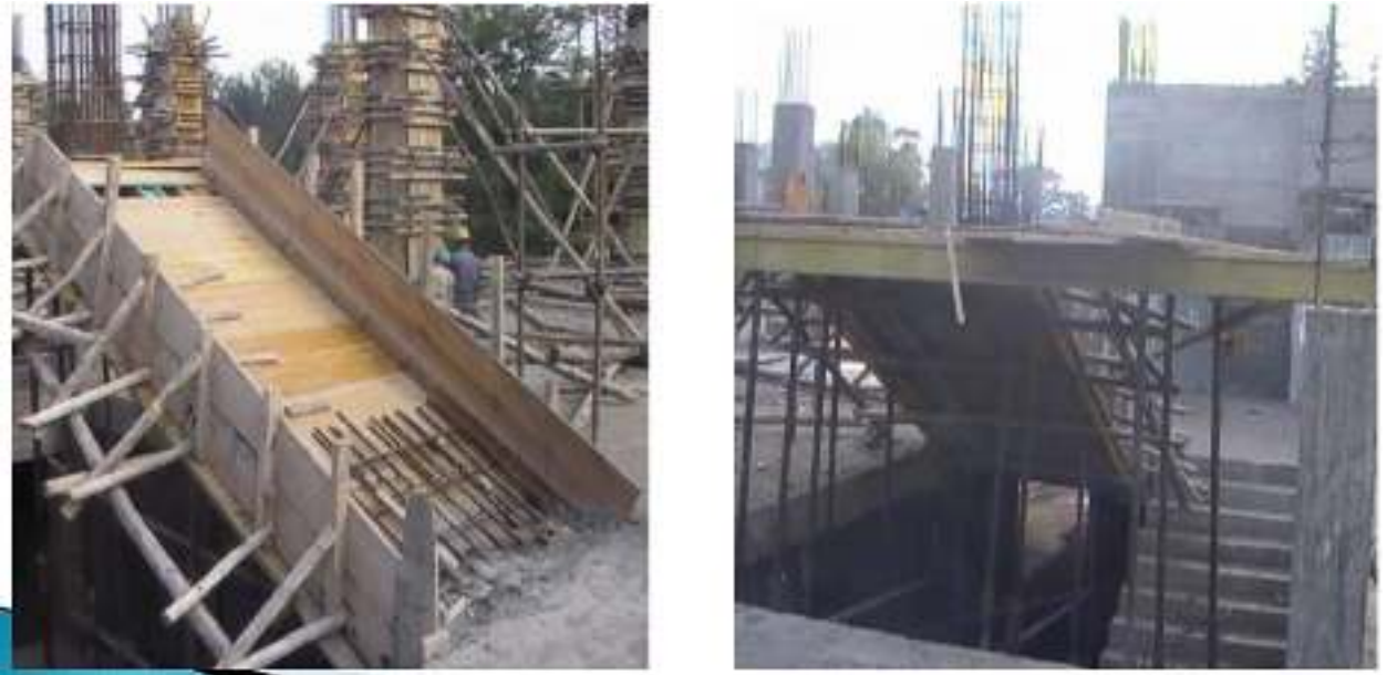
Fig.1.25. Timber stair formwork
