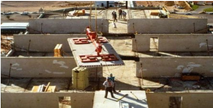
Fig.2.17. Placement of Hollow Core Precast Concrete Slab on Walls
