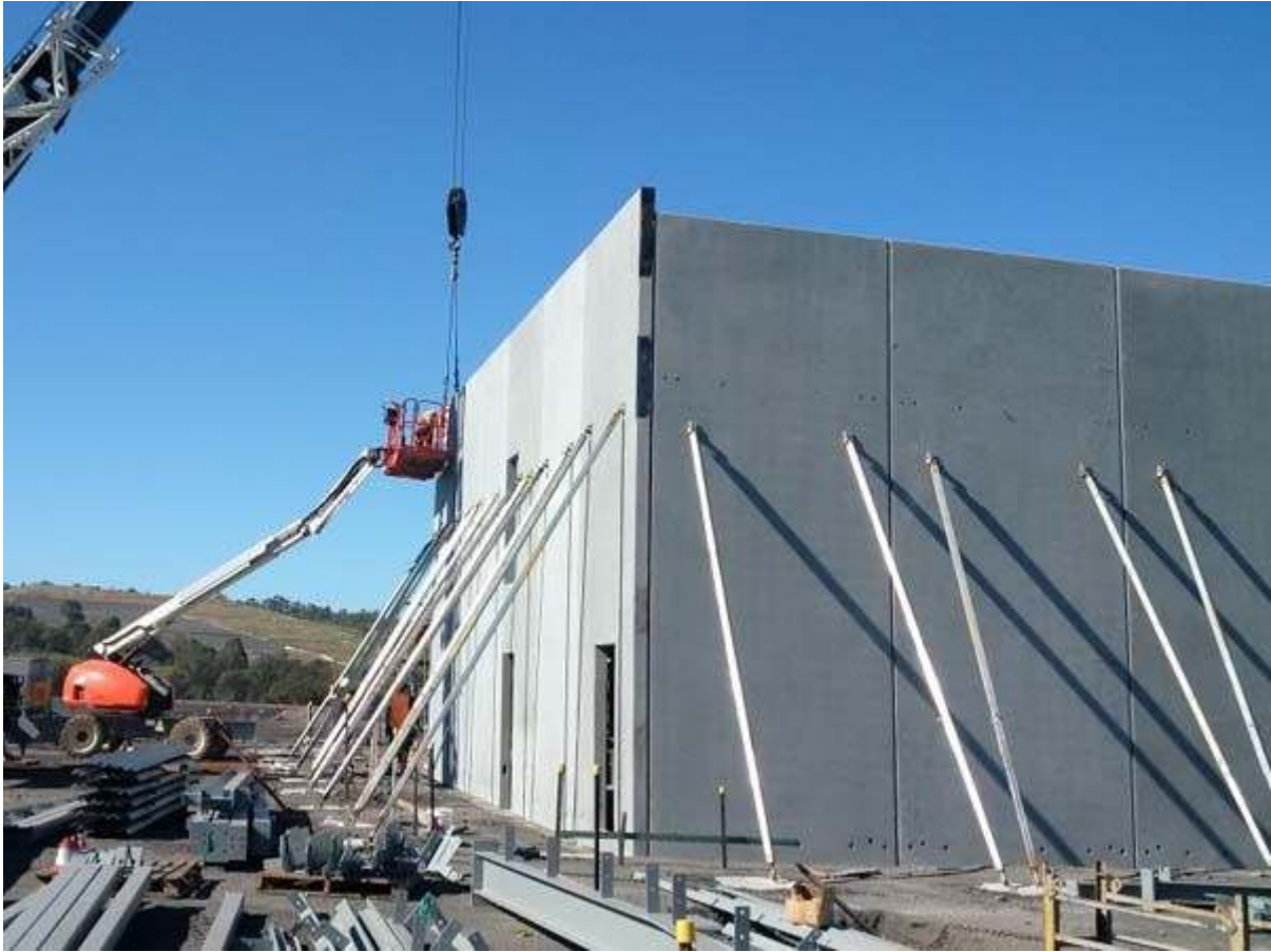
Fig.2.15. 2.Erecting temporary prop
