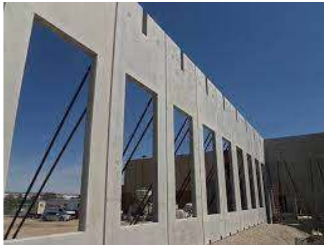
Fig. 3.1b. Concrete cladding panels
