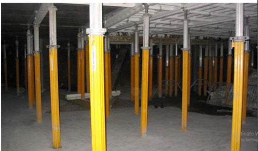
Fig.1.21. Steel Form Work for Slab
