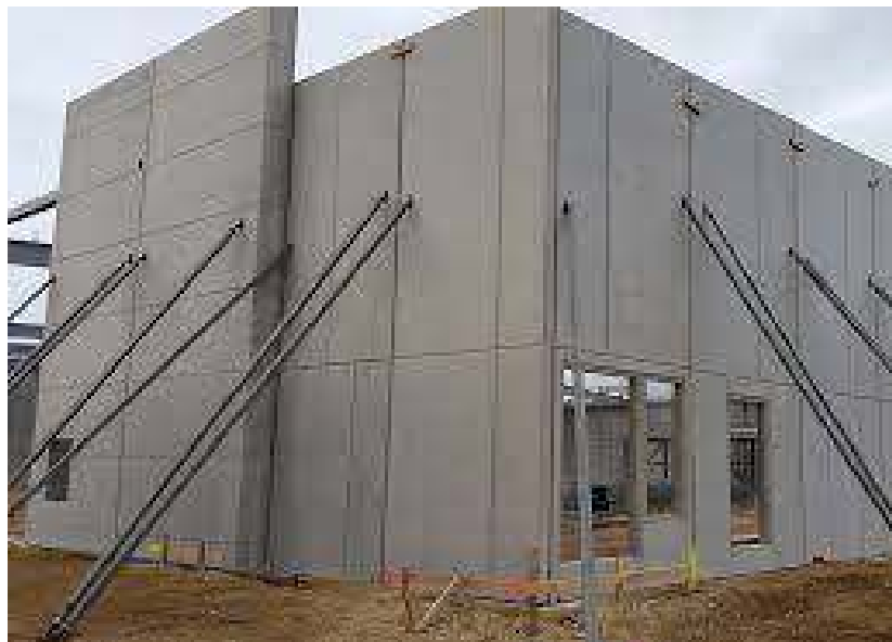
Fig.2.15.1.Erecting temporary prop
