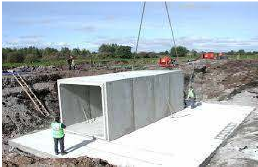
Fig. 2.8 fixing precast
