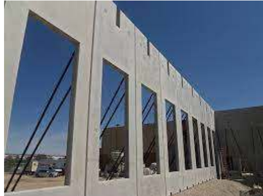
Fig. 3.3a: Fixing positioning for precast cladding
