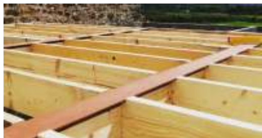
Figure 4.8 floor joists for straightens
