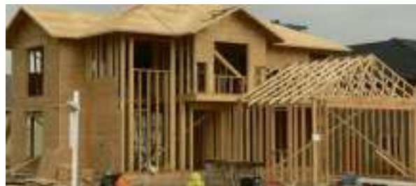
Figure 4.3 Rafters to Ceiling
