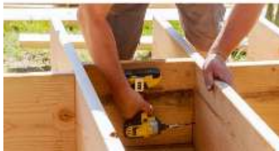
Figure 3.9 fixing beares
