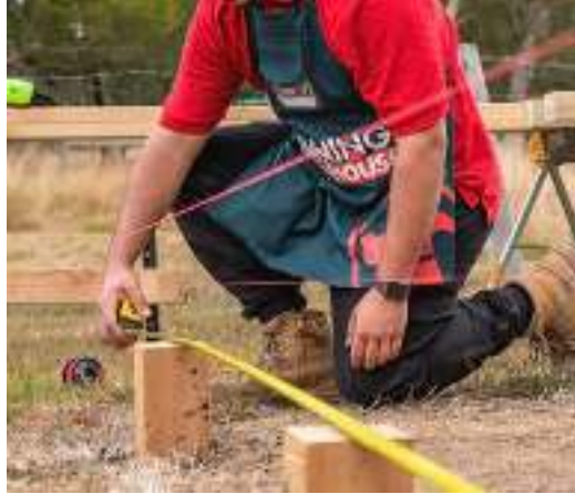
Figure 3.2 Mark and cut the stumps
