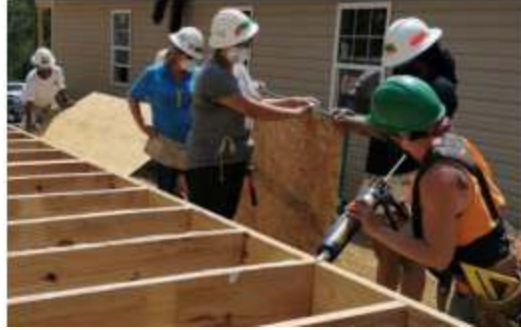
Figure 2.4 Floor Framing
