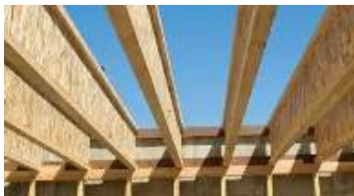
Figure 4.9 Flooring joists straightness
