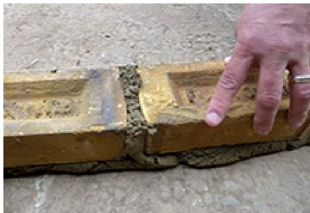
Fig. 3.13 laying the first
