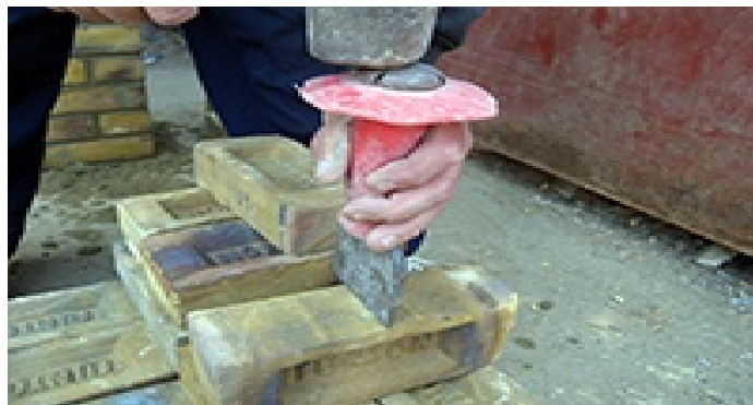
Fig.3.15 cutting brick
