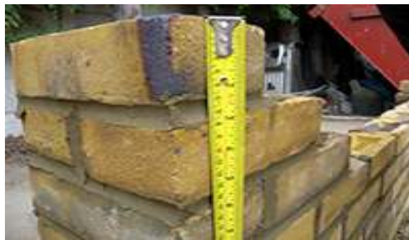
Fig. 3.17 checking mortar joints
