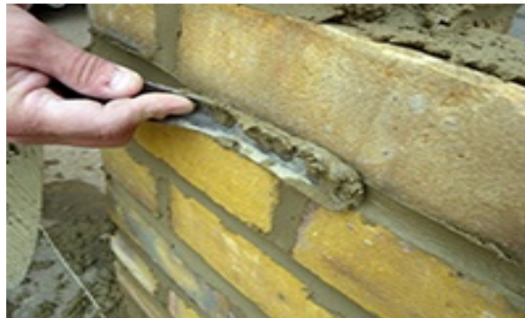
Fig. 3.21 finishing joints
