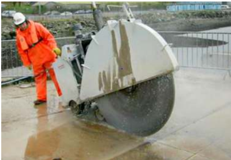
Figure 2.9 Concrete sawing method
