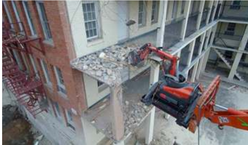
Figure 2.15 Selective demolition
