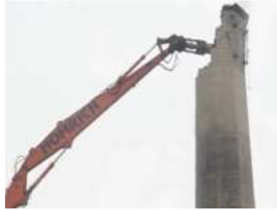
Figure 2.7 Pusher arm Technique
