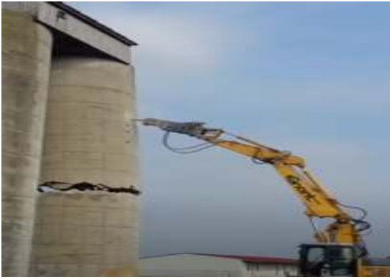
Figure 2.7 Pusher arm Technique
