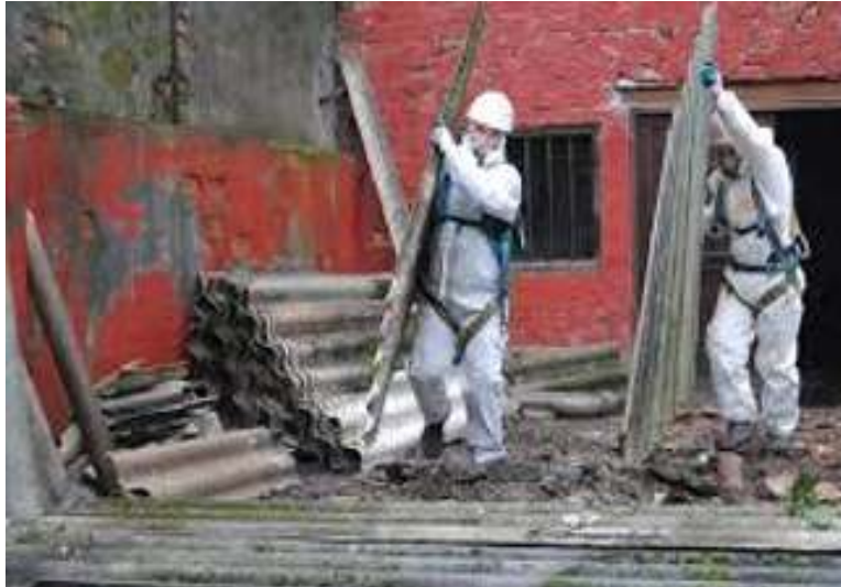
Figure 2.14 Removal of hazardous materials
