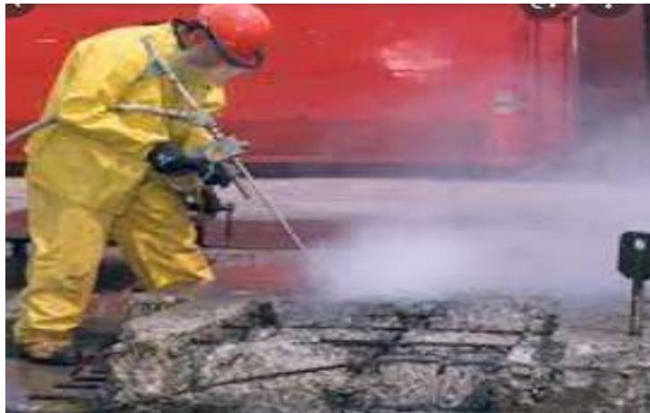
Figure 2.13 Pressure jetting
