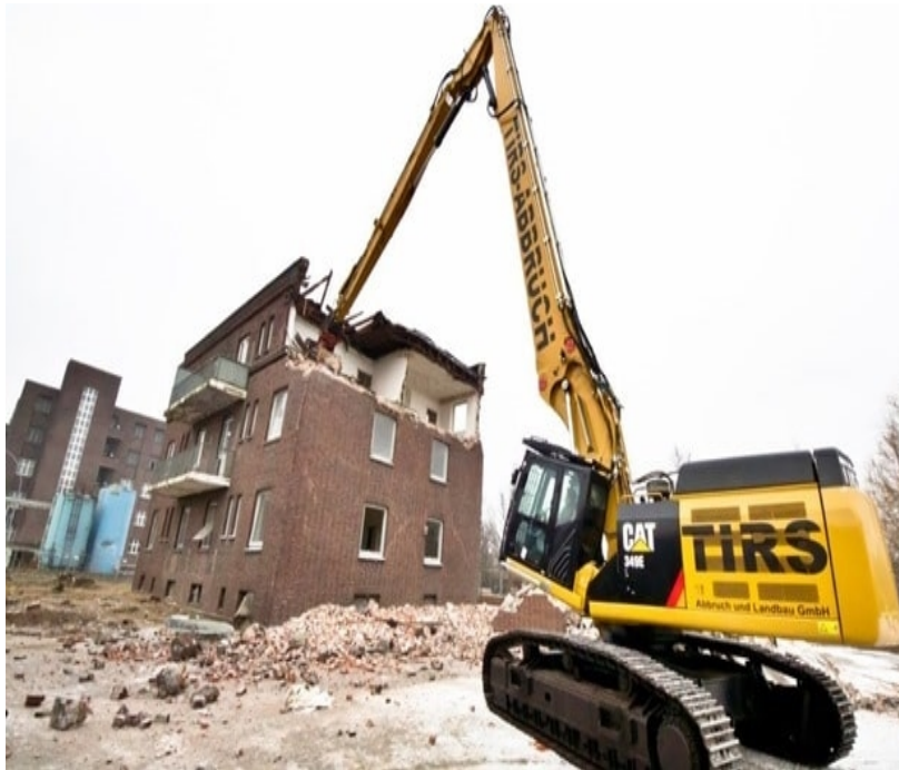
Figure 2.6 High Reach Excavators
