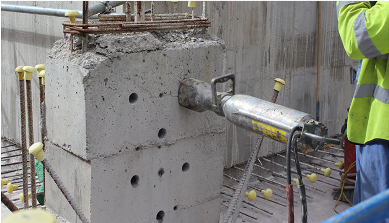
Fig.6.1. Bursting concrete
