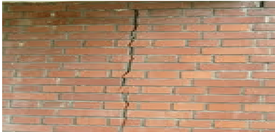
Fig.2.1 Carking Wall
