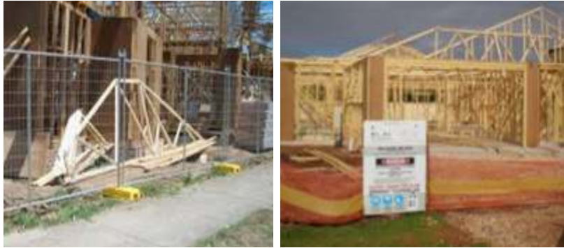
Fig.1.8 Signs and barricades to control access to a site
