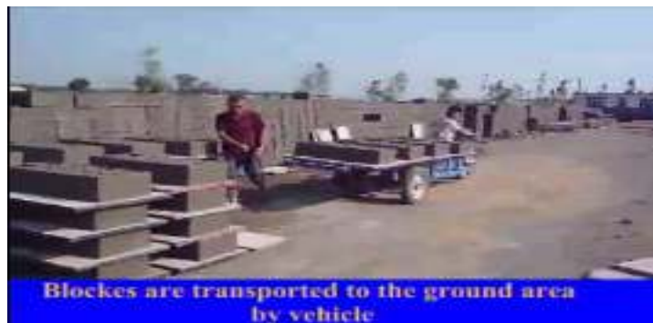
Fig.4.2Block Transported to stacking area to cure
