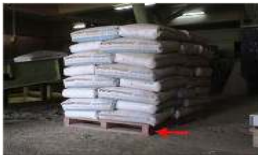
Fig.1.23 cement stacking
