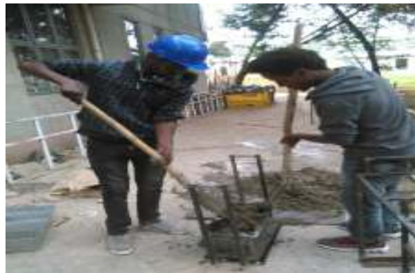
Fig.3.4 packing mold with mix
