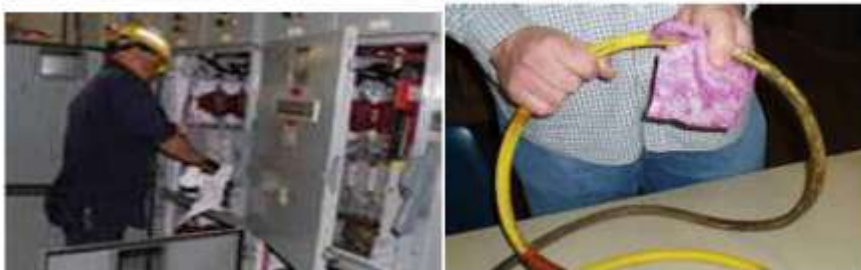
Figure 2.8 Clean out Look for tear/cut insulator
