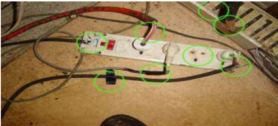
Figure 1.80 Hazardous socket
