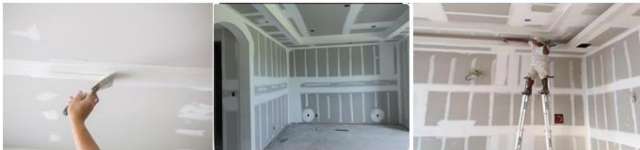
Fig 4.4 Application of Panel on wall and ceiling
