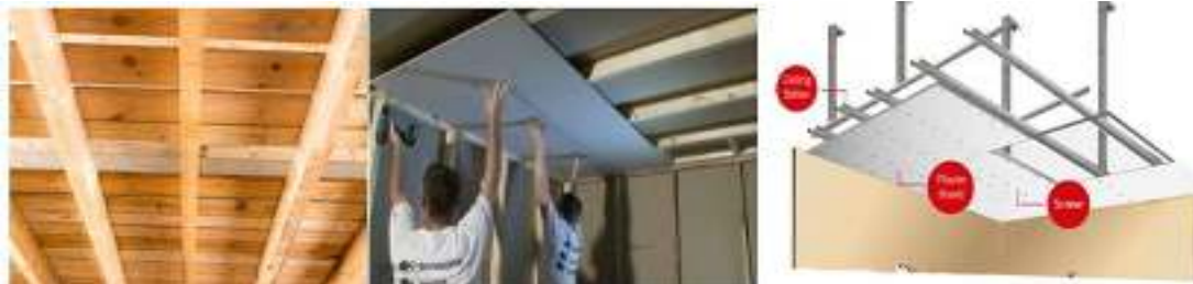
Fig 4.2 Application of Ceiling battens
