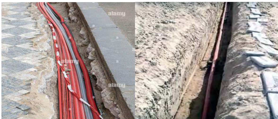
Figure 5.16 Direct Laying of Underground Cables
