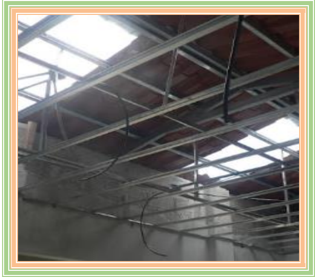
Fig.5.5. (b) Metal Studs for ceiling
