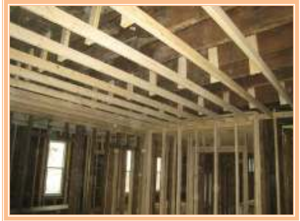
Fig.5.4. (b) Wooden Studs for ceiling
