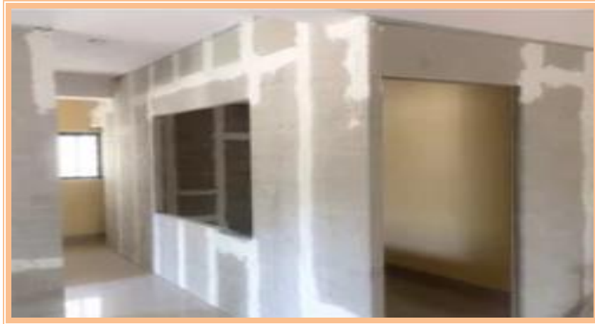
Fig.5.3. Partition Wall System
