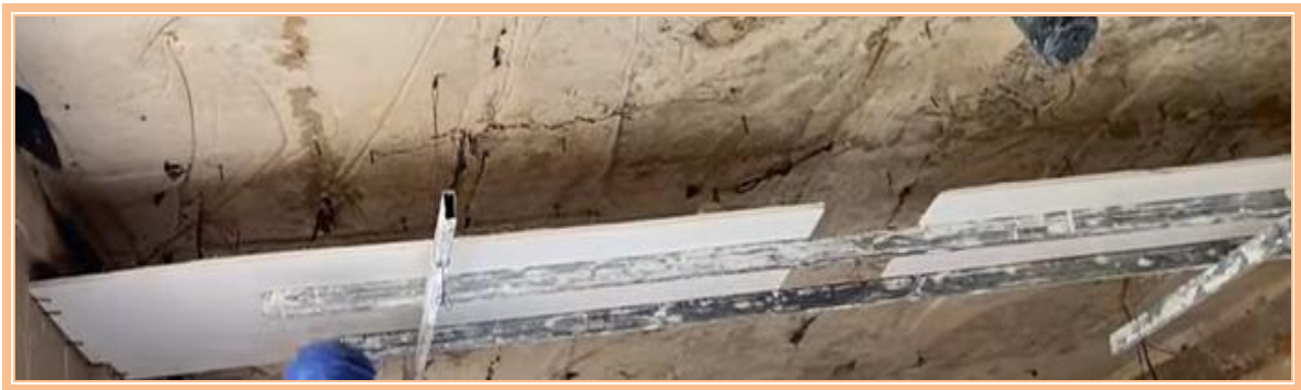
Fig 5.7. Place gypsum boards on the straight edge
