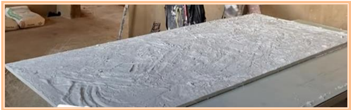
Fig:3.7. Demoulding Fiber gypsum board
