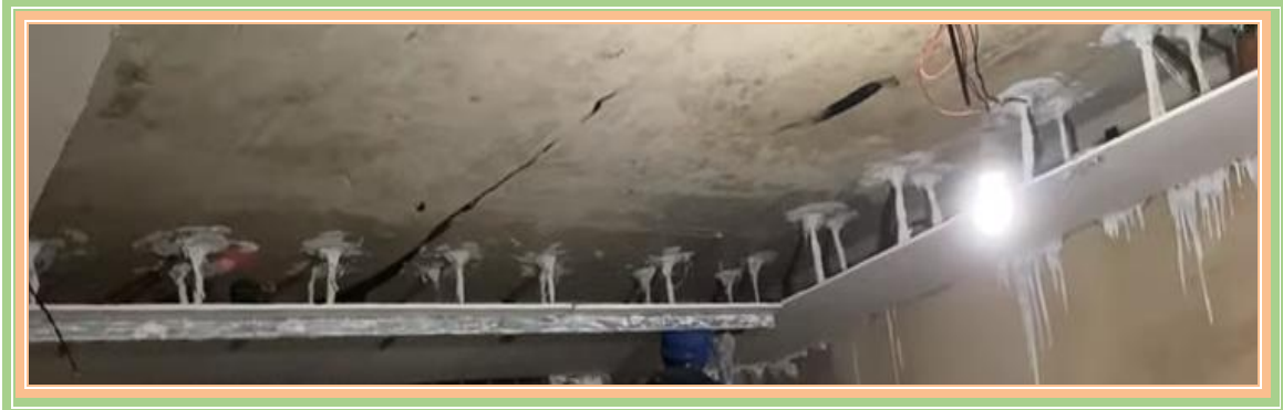
Fig 5.8. Hang the gypsum boards
