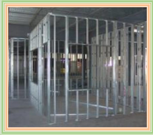
Fig.5.5. (a) Metal Studs for wall
