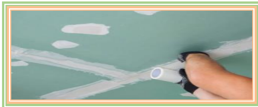
Fig 5.7. Joint Treatment
