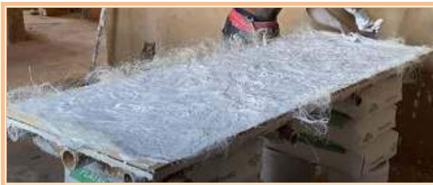
Fig:3.6. Spreading the Fiber of First Layer
