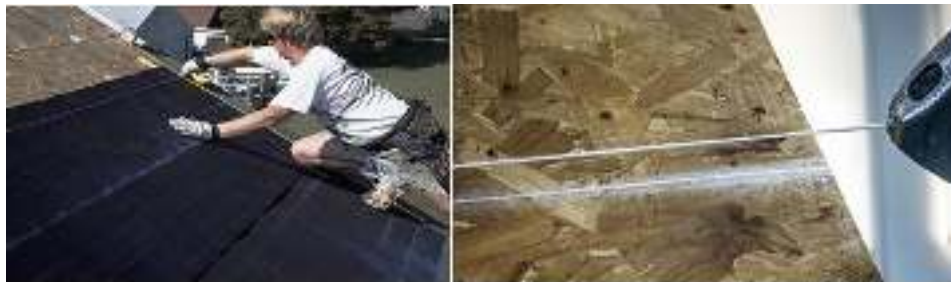
Figure 1.7 Chalk lines for roof work
