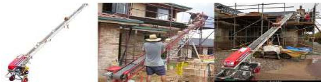
Figure 1.10 Elevators for roof work
