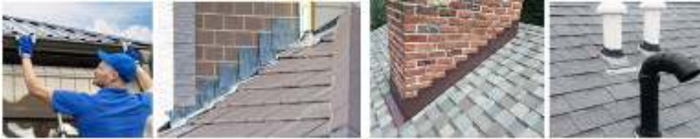
Figure 1.22 Application of flashing for roof
