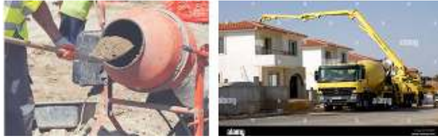
Figure 1.9 Concrete mixers for roof work
