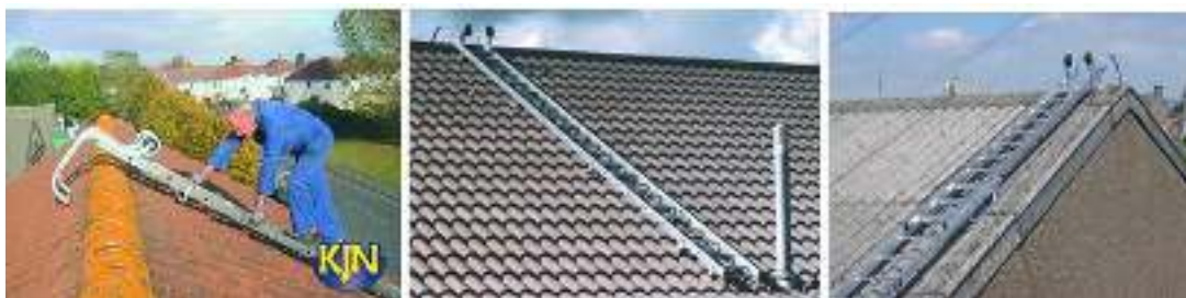
Figure 1.15 Ladders for roof work
