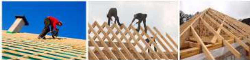
Fig 3.2 Battens Fixing
