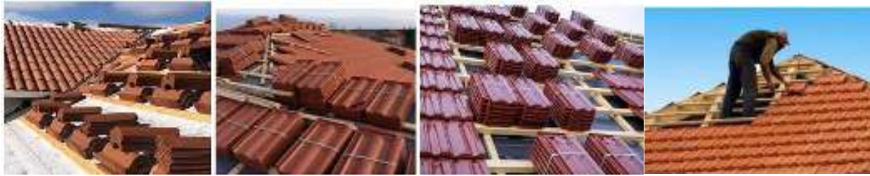
Fig 4.1 Loading tiles to roof
