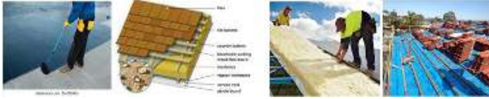
Figure 1.22 Application of sarking materials for roof
