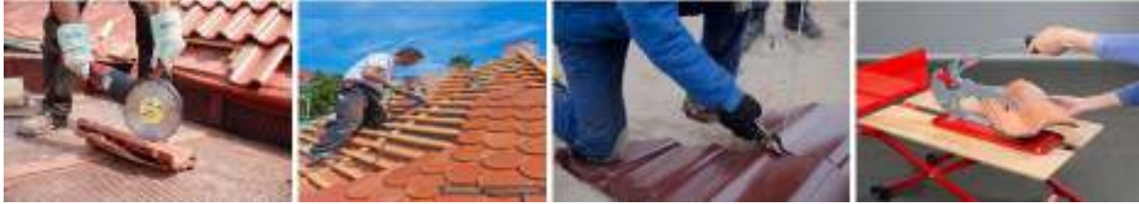
Fig 4.2 Roof tile cutting
