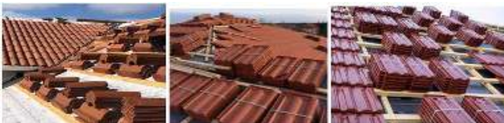
Figure 1.23 Handling of roof materials
