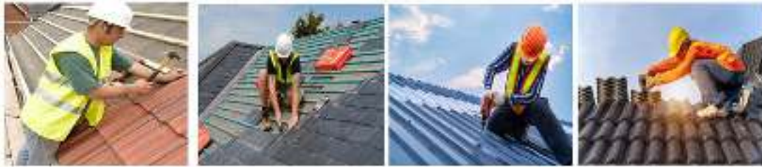
Fig 4.3 Securing tiles to roof
