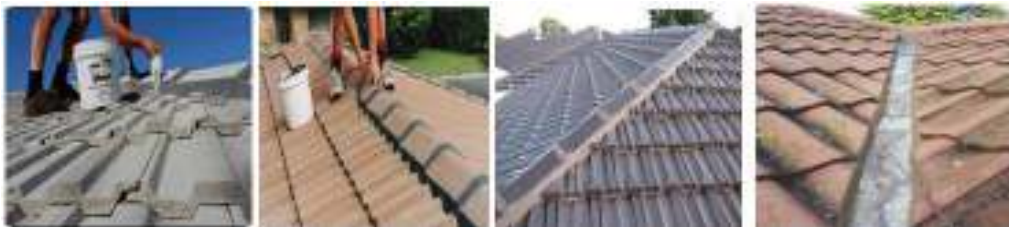
Fig 4.5 Pointing roof tiles
