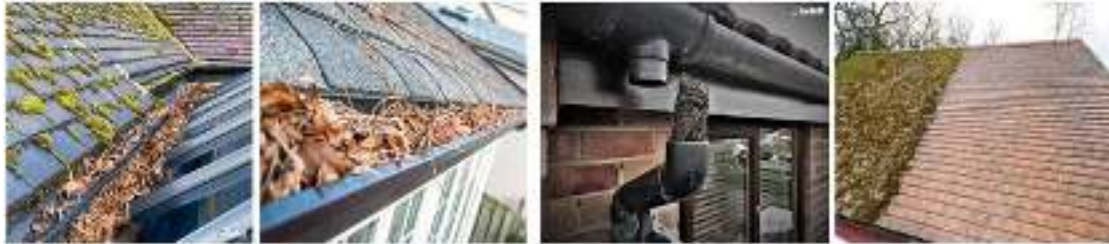
Fig 4.6 Clearing of roof
