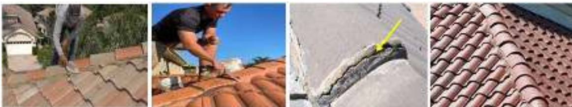
Figure 1.20 Pointing for roof work
