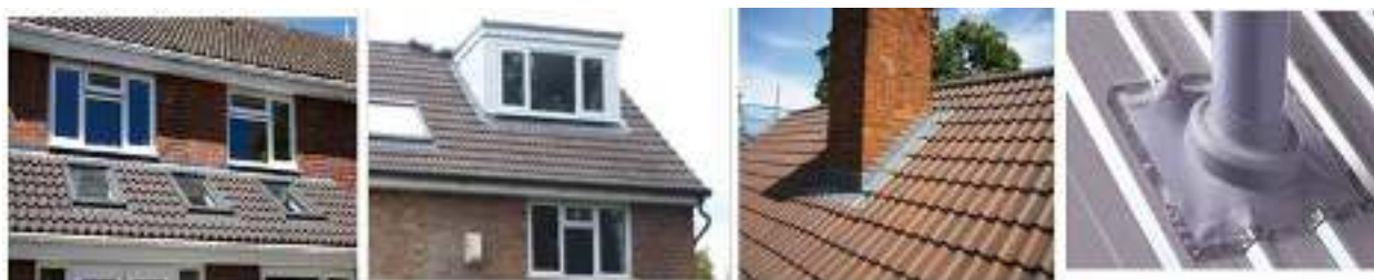
Fig 5.1 Openings on roofs
