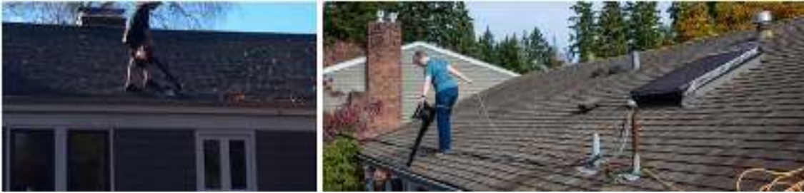
Figure 1.4 Blowers for roof clearing
