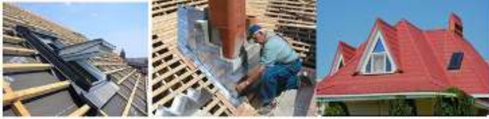
Fig 5.2 Application of weather proofing around roof openings
