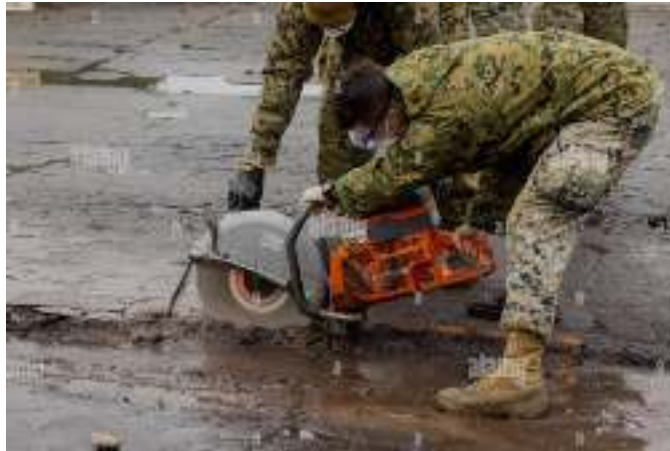
Figure 0-8 Cutting out damaged sections
