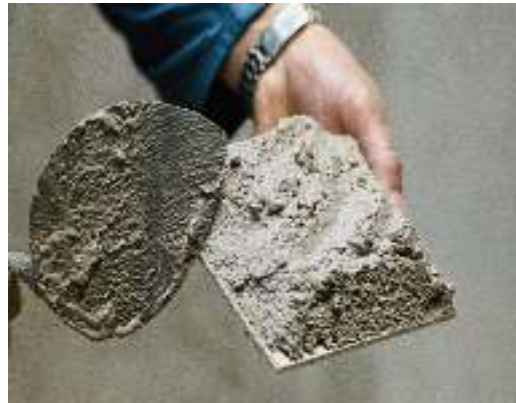
Figure 2.5 Thick Bed Mortar Applied on curved surface Tile
