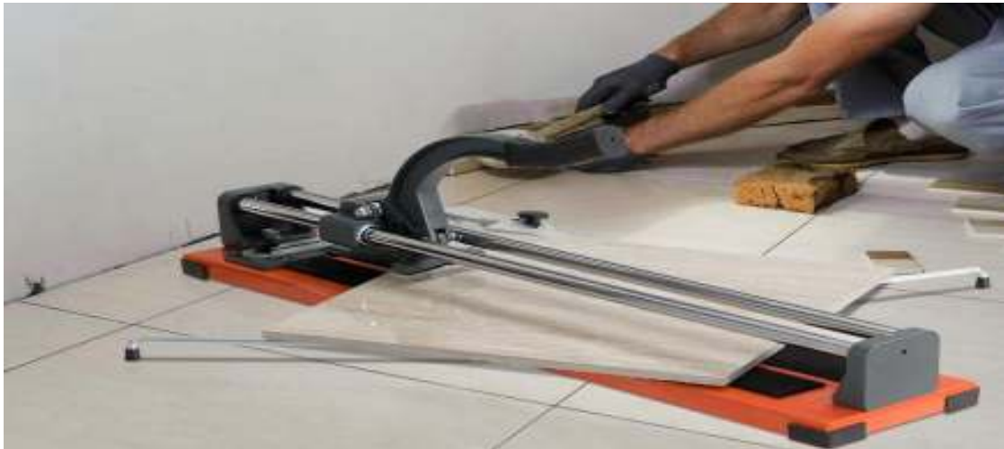
Figure2.3 tile cutting process
