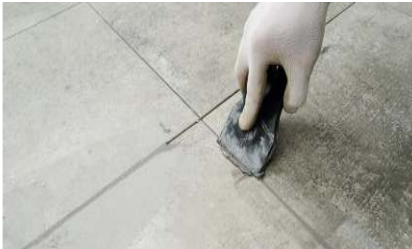
Figure2.7Seal the grout process
