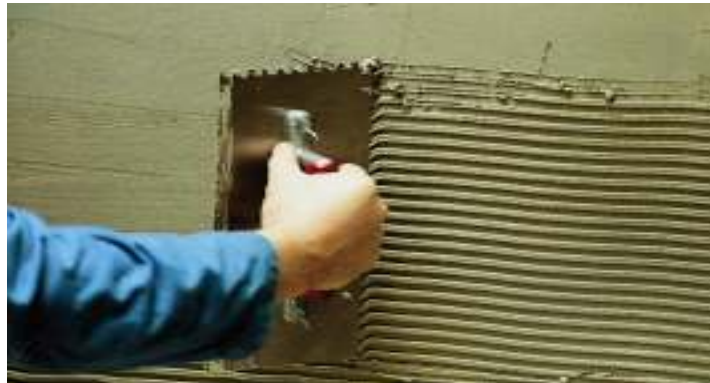
Figure 2.4 Application of thin bed mortar on a curved wall
