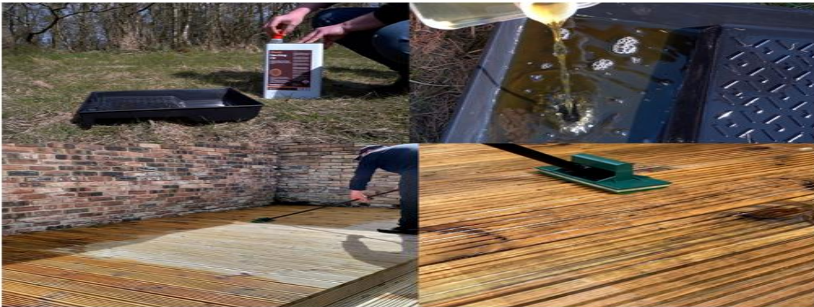
Figure 4-1 Applying clear timber finishing
