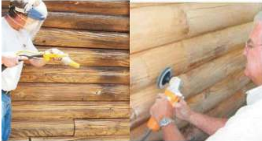
Figure 2-12 Stripping Existing Stained or Finished Surfaces
