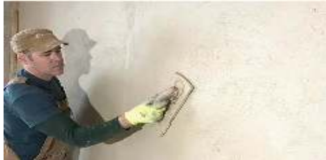
Figure1.2 lime plastering surface
