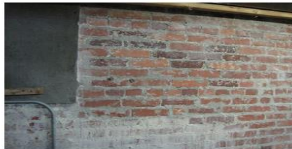
Figure2.2 brick background surface
