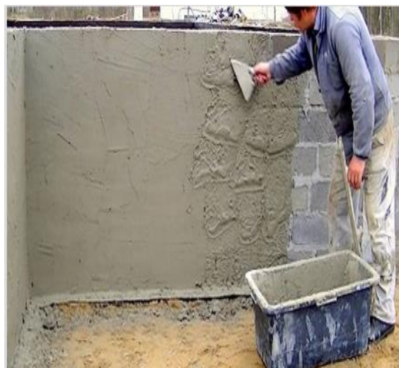
Figure4.13 first coat or single coat plastering
