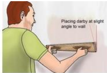
Figure4.7 placing darby at right angle to wall
