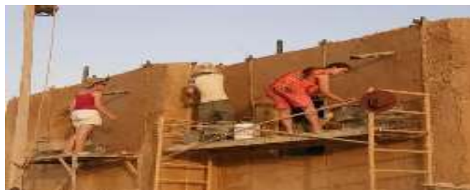
Figure1.3 mud plastering surface
