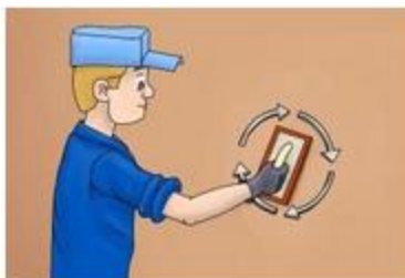
Figure4.8 use float plaster
