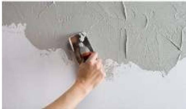
Figure1.5 Gypsum plastering wall
