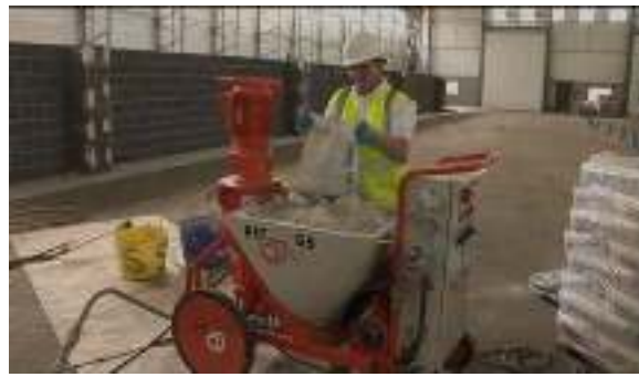
Fig 2.1 Mixing of mortar by plaster projection machine
