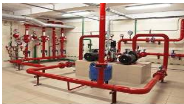
Figure 3.1: pipe support and hanger
