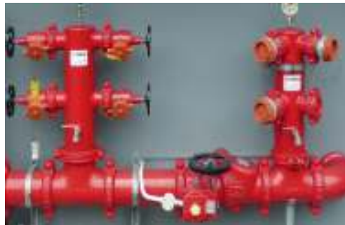
Figure 3.8 Fire hydrant
