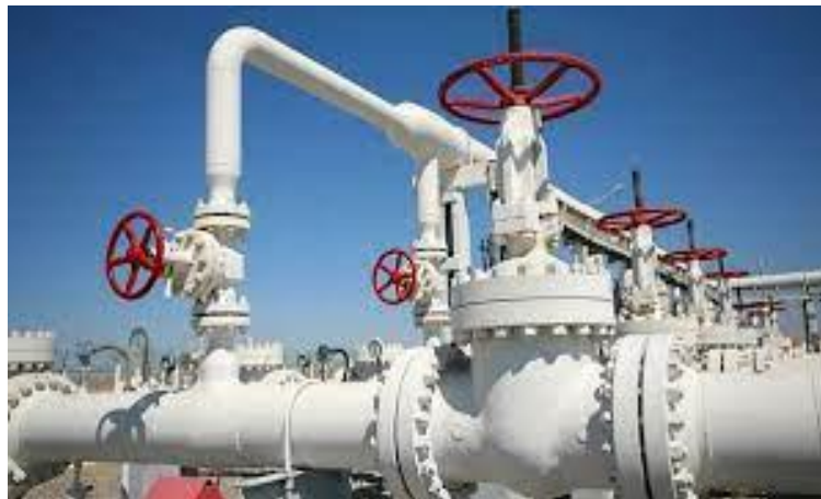
Figure 3.10 flanged valve
