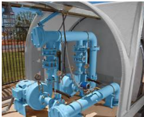
Figure 1.8 Municipal water supply
