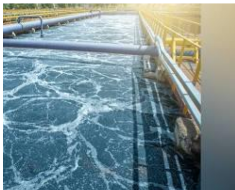
Figure 1-8 Water treatment aeration
