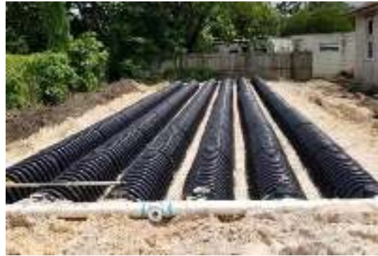
Figure 1-4 drain field system
