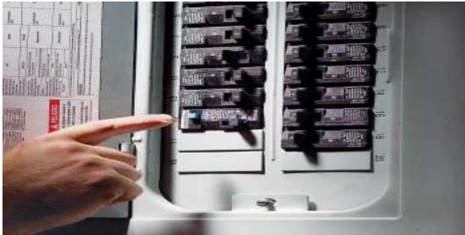
Fig 22. Replace Circuit breakers
