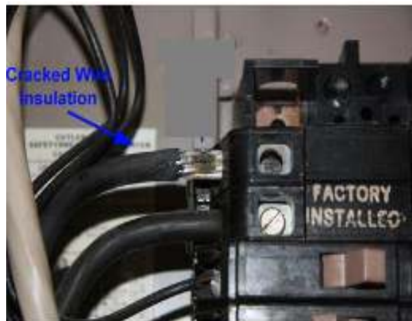
Fig 8. Loose Connections
