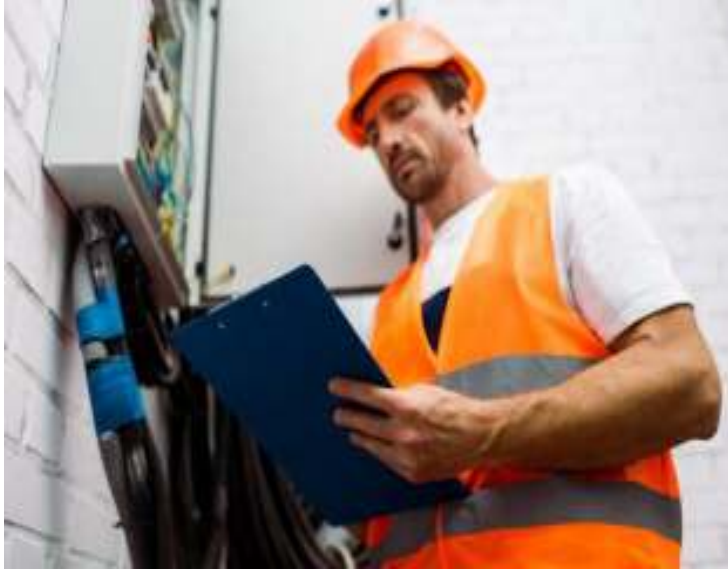
Fig 7. visual fault inspection
