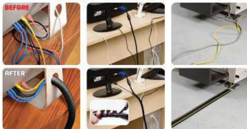
Figure4. 7 Cable management before and after in office
